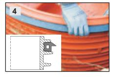
Install a gasket Ø1000 in the lowest groove on the outside of the ring. The groove should be thoroughly cleaned before gasket installation.
