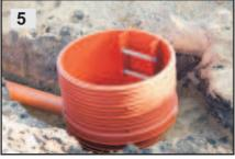
Lubricant should be applied onto a gasket Ø1000 before jointing with another manhole section. Products approved for rubber gaskets and plastic should be used. Note! If there are no rings of diversified heights on a building site, rings of standard heights may be cut. Rings may be cut only at marked places every 25 cm.
