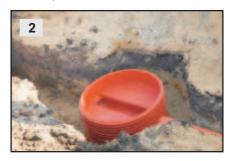
Place a base unit on a prepared earlier sand bedding and level it and then connect sewage pipes to the chamber A place where a manhole is located should be lowered by approximately 10 cm. Connect sewage pipes.
