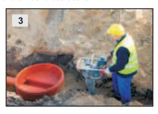
Fill up the trench with preliminary backfill (10 cm above the pipe level). Compaction should be performed manually, in layers every 15 cm or with light mechanical equipment (each layer up to 30 cm). Base unit 1000 should protrude above the backfill level.
