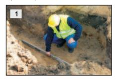
Prepare a trench in an inspection chamber location removing large and sharp-edged stones. On the trench bottom prepare bedding composed of compactable soil, preferably sand (coarse- medium- or fine-grained) of minimum 10 cm thickness An inspection chamber zone should include an area of at least a 30 cm wide strip around the chamber.
