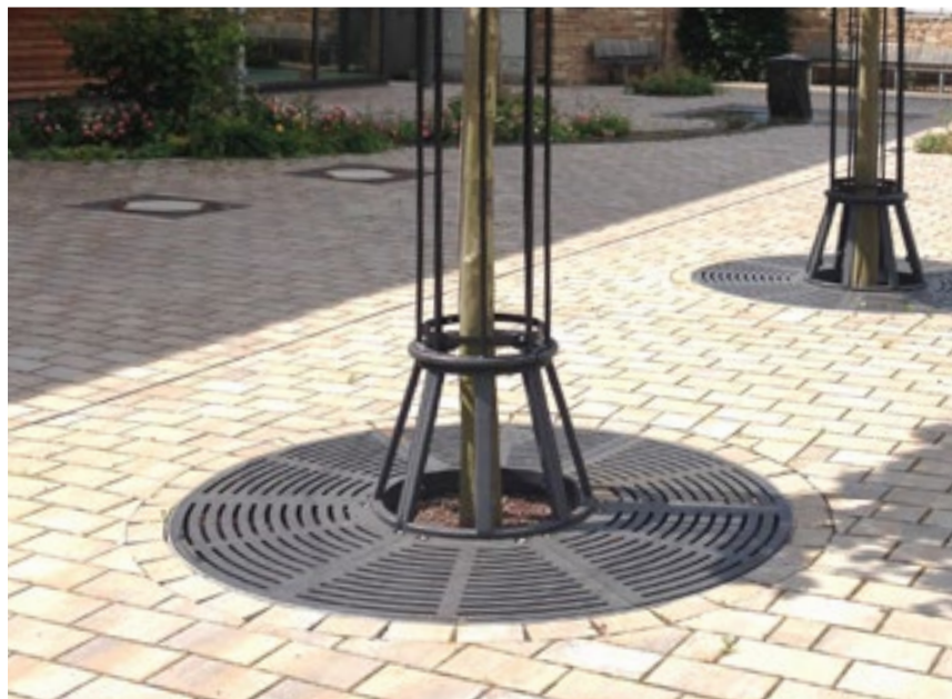
Collision protection with tree guard upper part - from page 28
